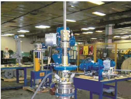
Tie-in equipment assembly and test area
